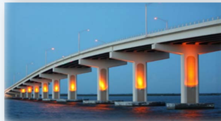
- Lighting for Max Brewer Bridge & Pier
