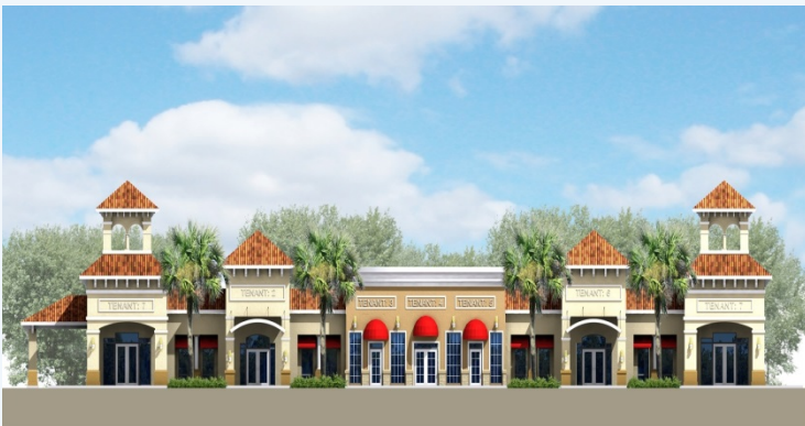
- Shoppes at Southwinds Retail Office Building
